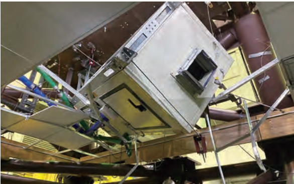
Experiments conducted in collaboration with Japan and Korea confirmed that suspended equipment with inadequate seismic design can pose serious risks to life safety.
